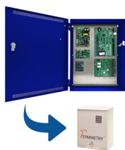
Replaced 30 AMAG proprietary panels with BluBOX Open Platform
